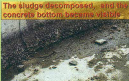
The sludge decomposed, and the concrete bottom became visible
